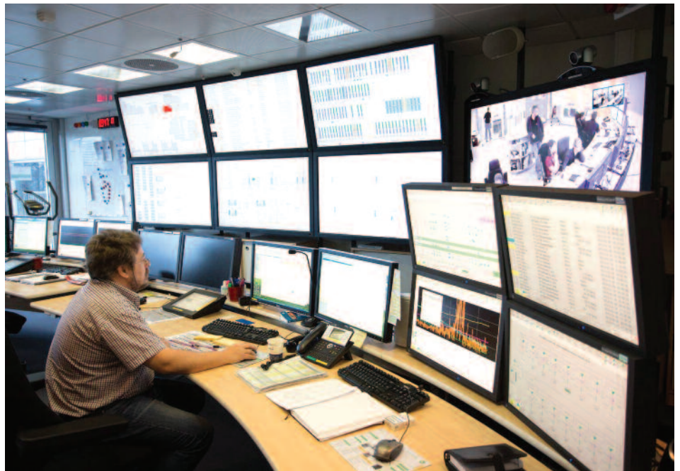
The Valhall onshore control room
